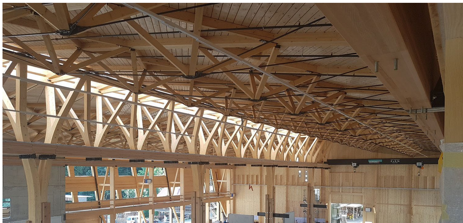
Fig. 3: Roof beams and crane tracks made of Swiss beech wood (Fagus Suisse)
