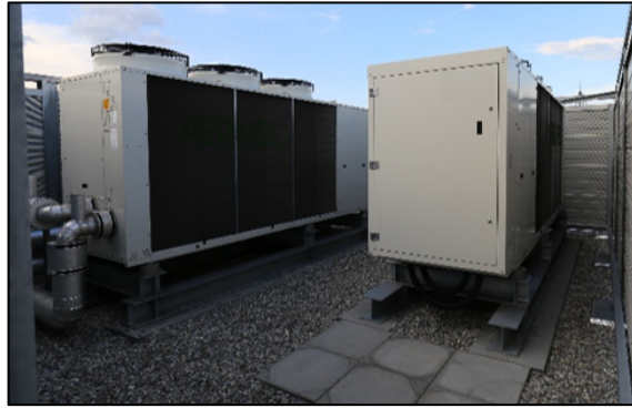
Monovalent system – Large industrial HP units
