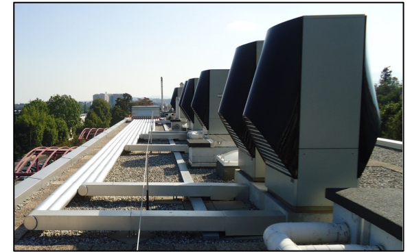
Bivalent system – Small standardized HP units
